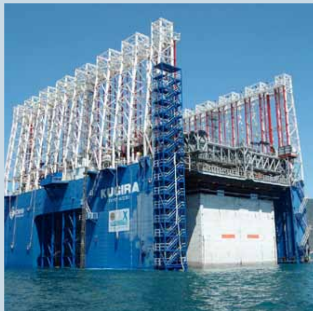
The Kugira floating dock (right) will manufacture all caissons that will be used in the construction of the Açú Shipyard.
