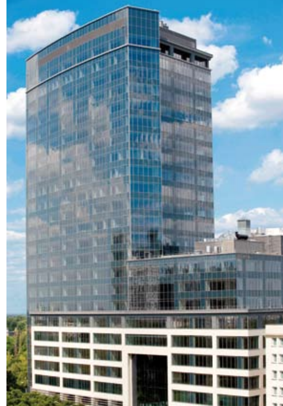
Facade of the 87m-high North Gate building, combining two types of glass.
