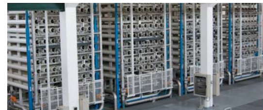
Example of membrane racks in the desalination plant in Jávea (Alicante).
